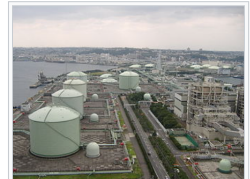
Regasification terminal of Tokyo Gas in Yokohama
