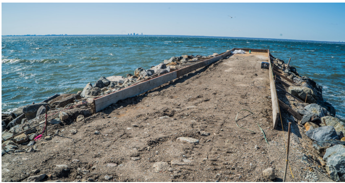
Webb's Pier in the beginning phases of reconstruction
