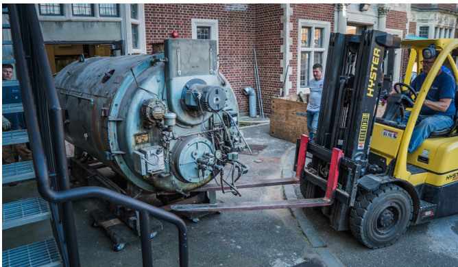
One of the old boilers being taken out
