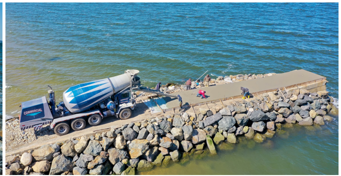
Cement truck carefully drives down the pier
