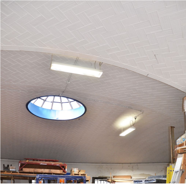
The historic Guastavino tile archway ceilings in the garage.
