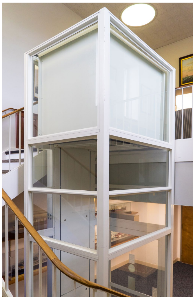
Right: ADA compliant vertical platform lift linking the college's newly constructed Couch Academic Center (CAC) to the historic STH.
